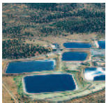
Commercial evaporation pits that accept fluids from independent truckers for a fee.
