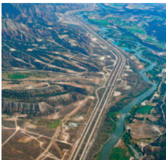
Drilling activities along both sides of the Colorado River.
